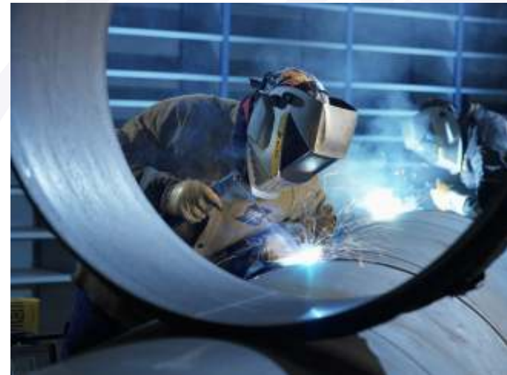
SMAW welding of pressure vessels
