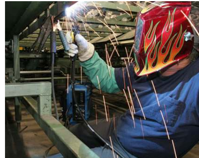
WELDING OUT OF POSITION
